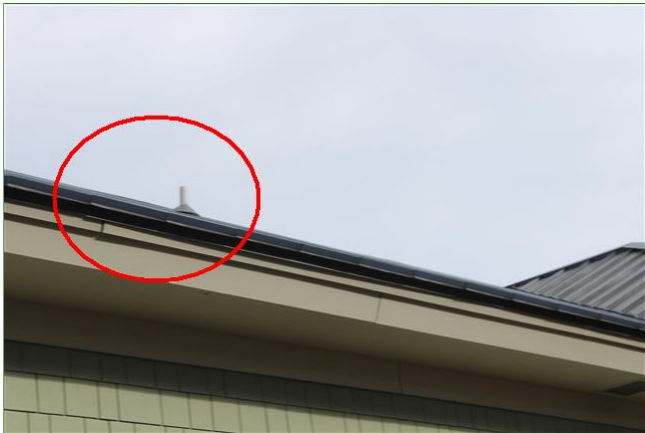
1.2 Item 1(Picture) Plumbing Vent with Boot
