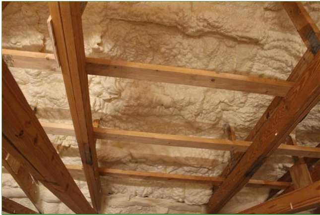
1.7 Item 3(Picture) Foam Insulation
