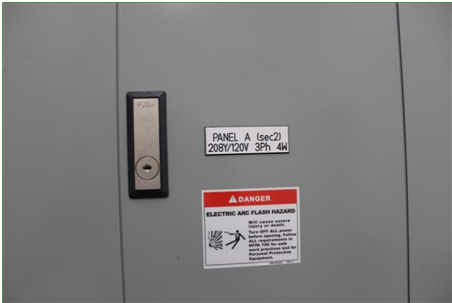
6.0 Item 4(Picture) 3 Phase/4 Wire Electrical Service
