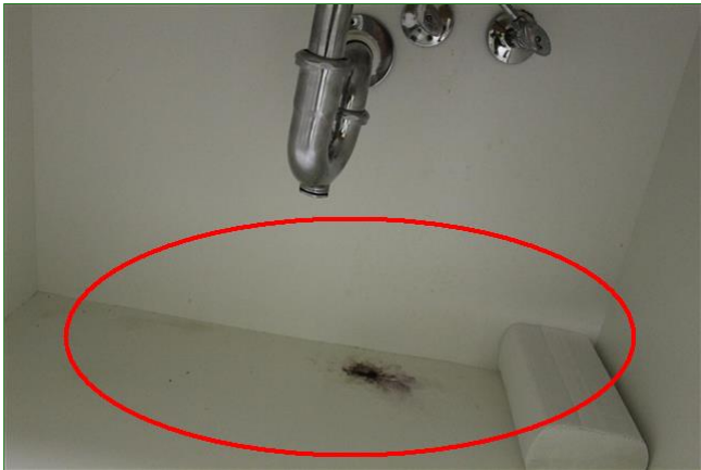
5.5 Item 1(Picture) Plumbing Inspected - Prior Water Damage - Area Was Dry
