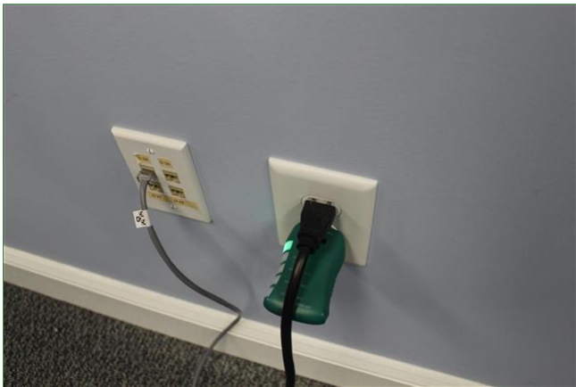
8.8 Item 3(Picture) Outlet Tested
