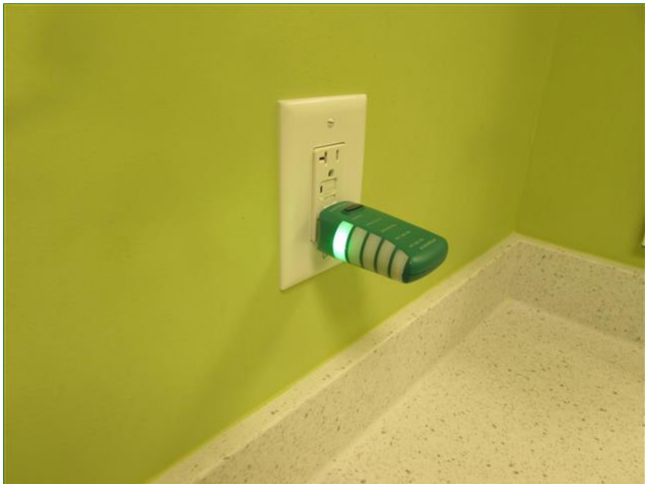
5.3 Item 3(Picture) Outlet Tested
