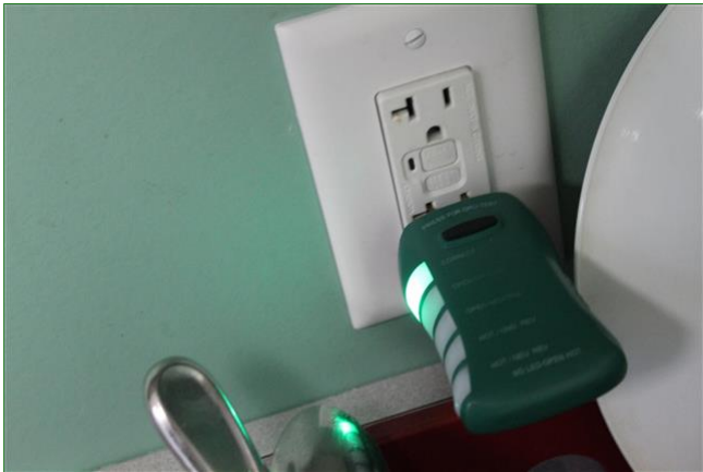
7.7 Item 1(Picture) Outlet Tested
