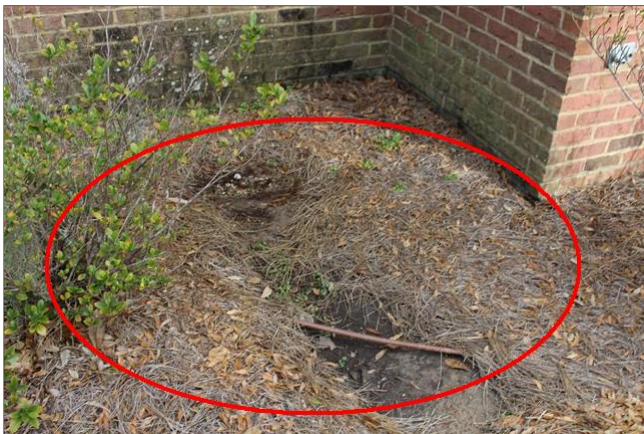
1.3 Item 4(Picture) Erosion from Water Collection Point
