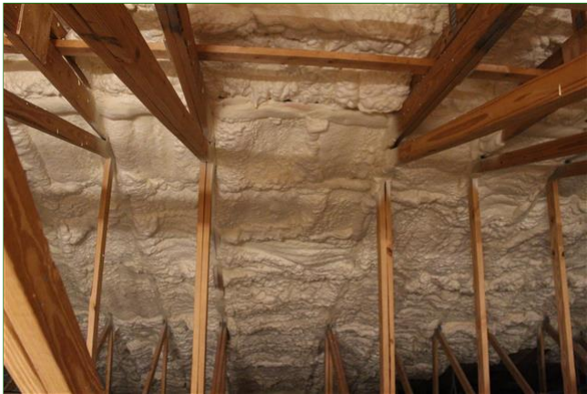
1.7 Item 4(Picture) Foam Insulation
