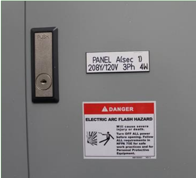
6.0 Item 3(Picture) 3 Phase/4 Wire Electrical Service
