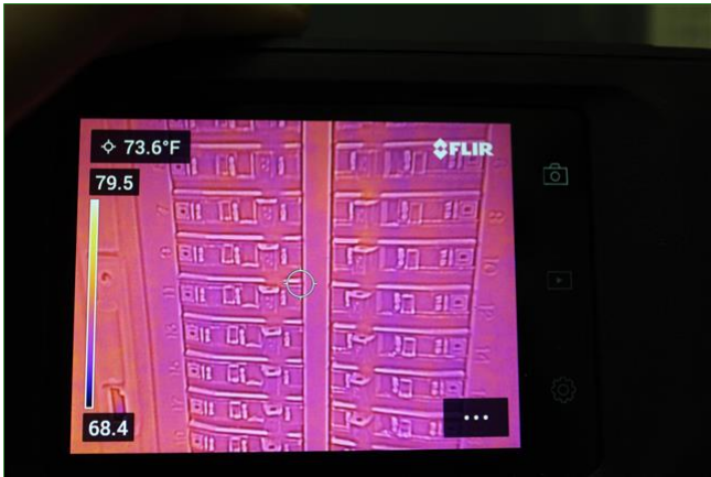
6.12 Item 5(Picture) Testing for Hot Spots
