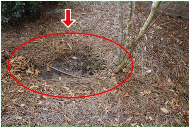
1.3 Item 2(Picture) Erosion from Water Collection Point
