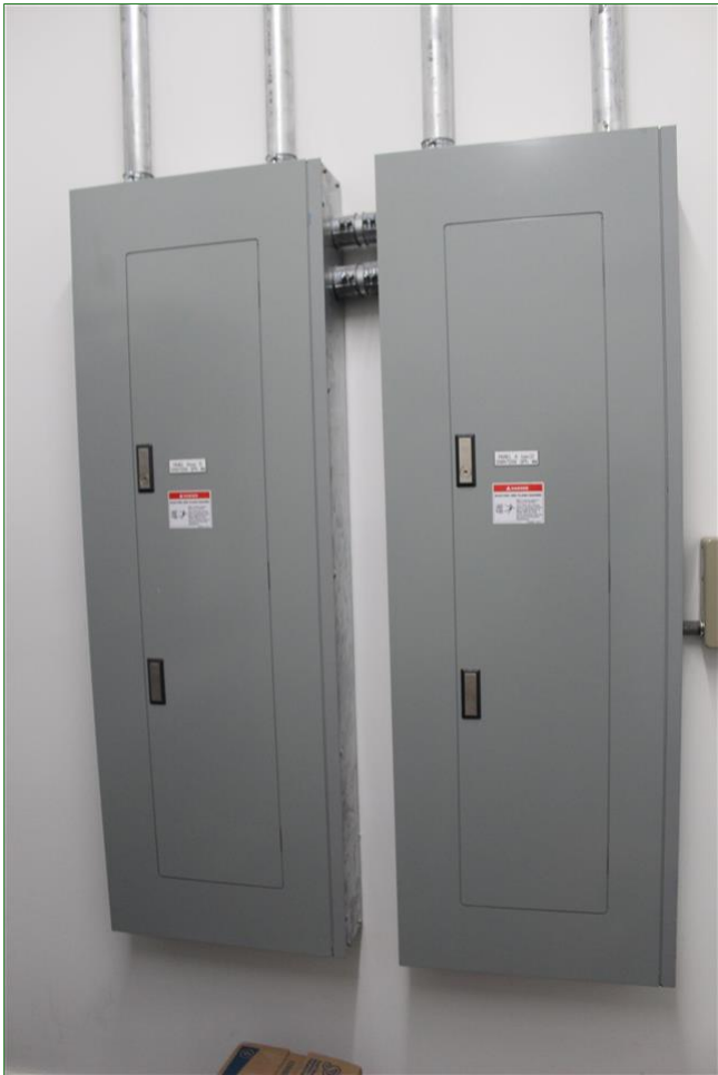
6.0 Item 2(Picture) 3 Phase/4 Wire Electrical Service
