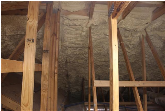
1.7 Item 5(Picture) Foam Insulation
