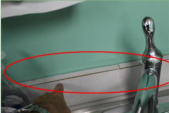
7.5 Item 6(Picture) Water Damage - Top of Back Splash
