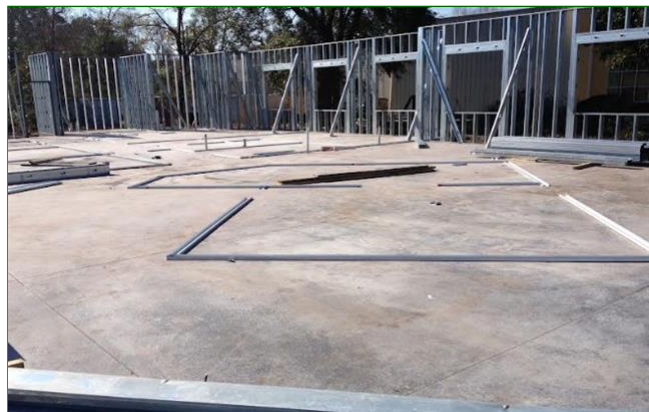
8.0 Item 1(Picture) Concrete Slab and Metal Studs
