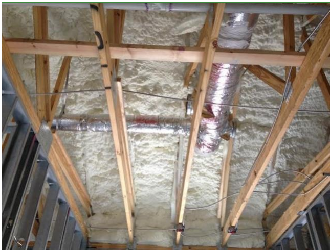
8.0 Item 4(Picture) Roof with Foam Insulation
