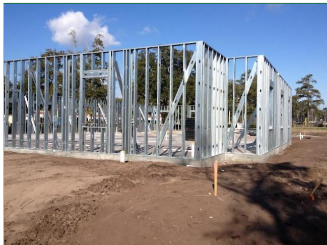
8.0 Item 2(Picture) Concrete Slab and Metal Studs
