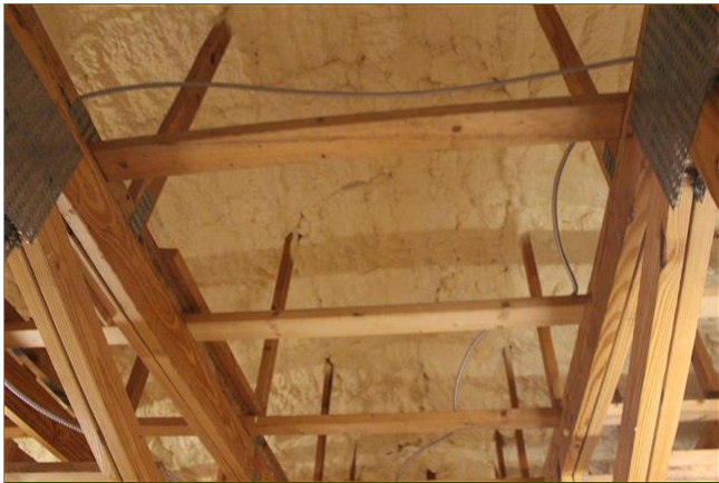
1.7 Item 2(Picture) Foam Insulation
