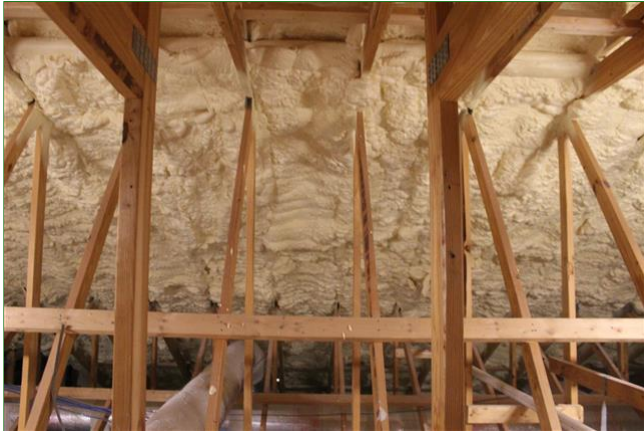
1.7 Item 6(Picture) Foam Insulation
