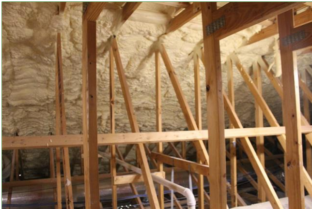
1.7 Item 7(Picture) Foam Insulation
