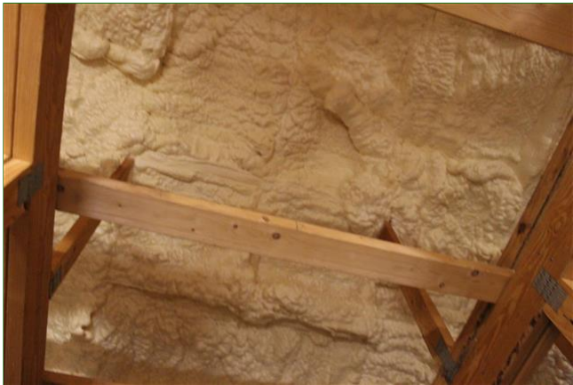
1.7 Item 1(Picture) Foam Insulation
