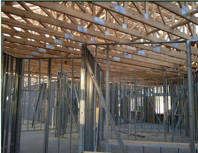
8.0 Item 3(Picture) Concrete Slab, Metal Studs and Roof Structure
