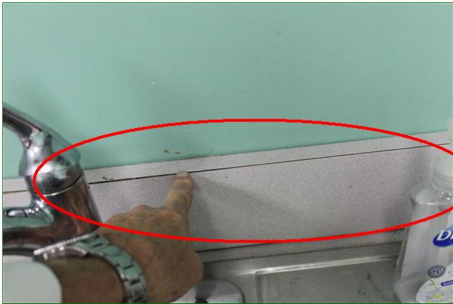
7.5 Item 7(Picture) Water Damage - Top of Back Splash
